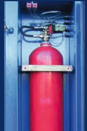
Complete containerised solutions including fire fighting system
